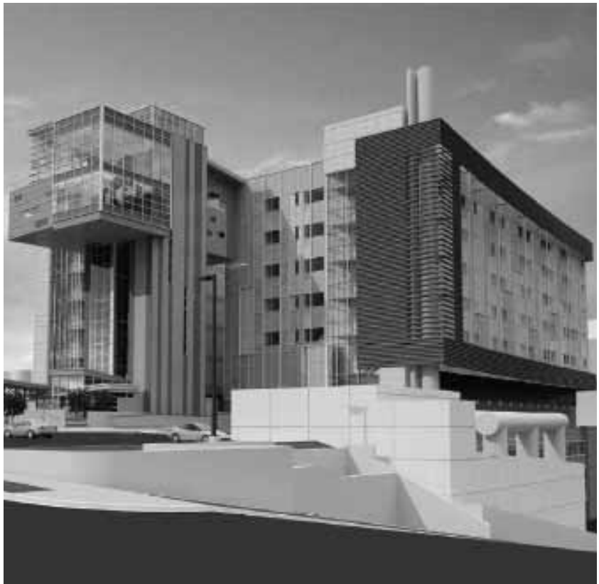
A computer-generated view of the Vertical Expansion from the corner of Irving Ave. and Adams St.
