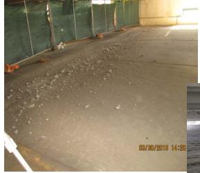
The contractor has to secure the next floor below the proposed work to protect people and vehicles from falling construction debris.
