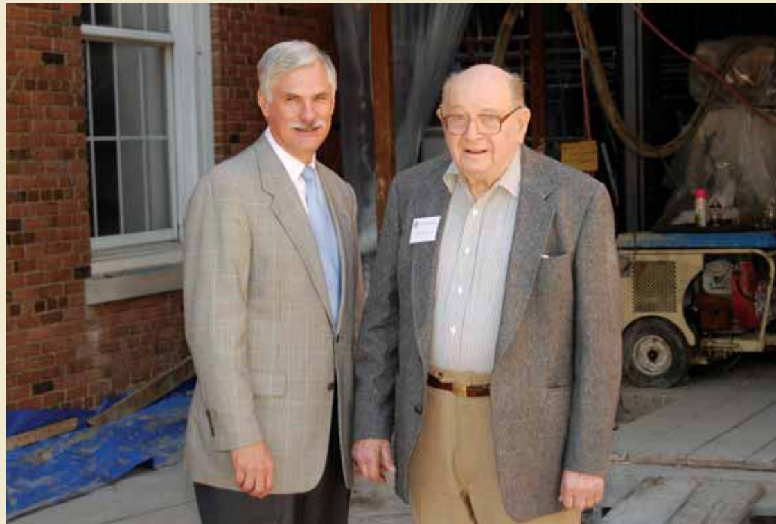
Construction of the Setnor Academic Building is on pace for completion in spring 2007. Jules R. Setnor, MD '35, (right) got a recent look at the building's progress with Upstate President David Smith, MD.
