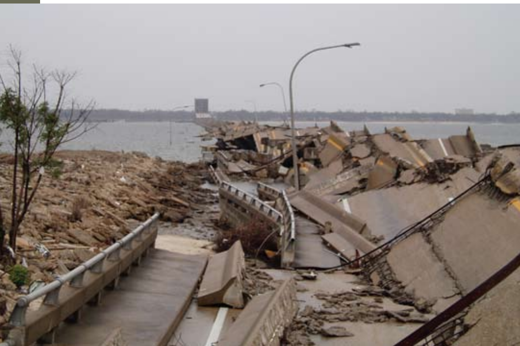
Above: New Orleans Biloxi Bridge in the wake of Hurricane Katrina, July 2006. Right: The Great Flood Commemoration, New Orleans, August 2006.
