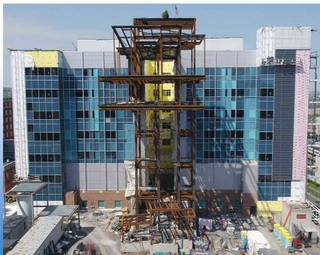
Construction photo taken May 2008.
