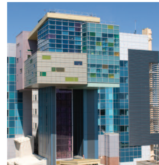
East Tower addition of Upstate University Hospital. Central projection is the "tree house" entrance to the top two floors which make up the newly opened Upstate Golisano Children's Hospital.
