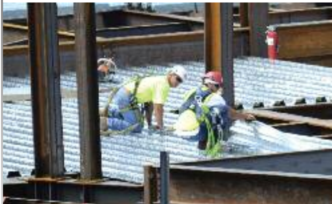
Top: Architect’s rendering of the Upstate Cancer Center, scheduled to open in 2013. Above: Steel workers from Rauli and Sons, Inc. of Syracuse install metal decking at the Upstate Cancer Center in July.
