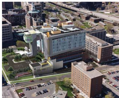
Figure 1: Aerial north view of the Vertical Expansion.
