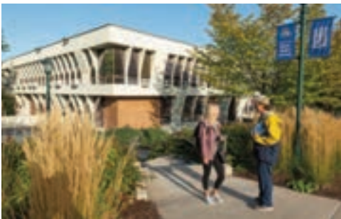
Campus Activities Building
