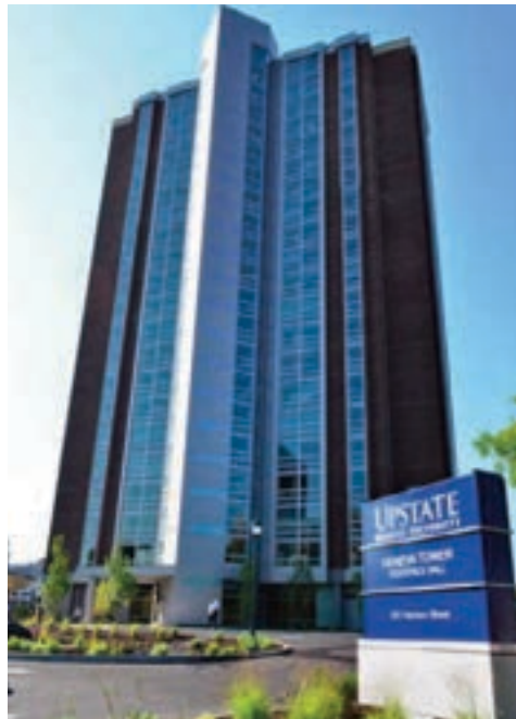
Geneva Towers, a residential facility
