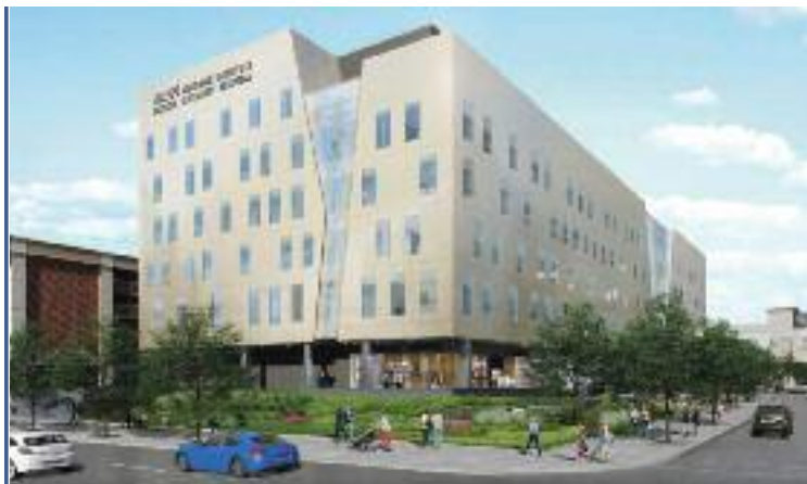
Construction has begun on the Nappi Longevity Institute, which will house an array of services.
