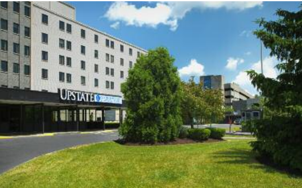
Upstate Community Hospital, a part of Upstate since 2011, is a suburban hospital four miles from the downtown campus.
